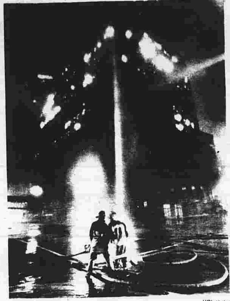
FIREFIGHTERS BATTLE THANKSGIVING NIGHT BLAZE. Minneapolis fire damage total: $91 million.
